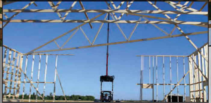
Telescoping boom extends beyond 21 feet
