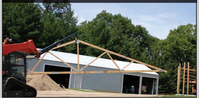
Securely transport and position materials at the job site
